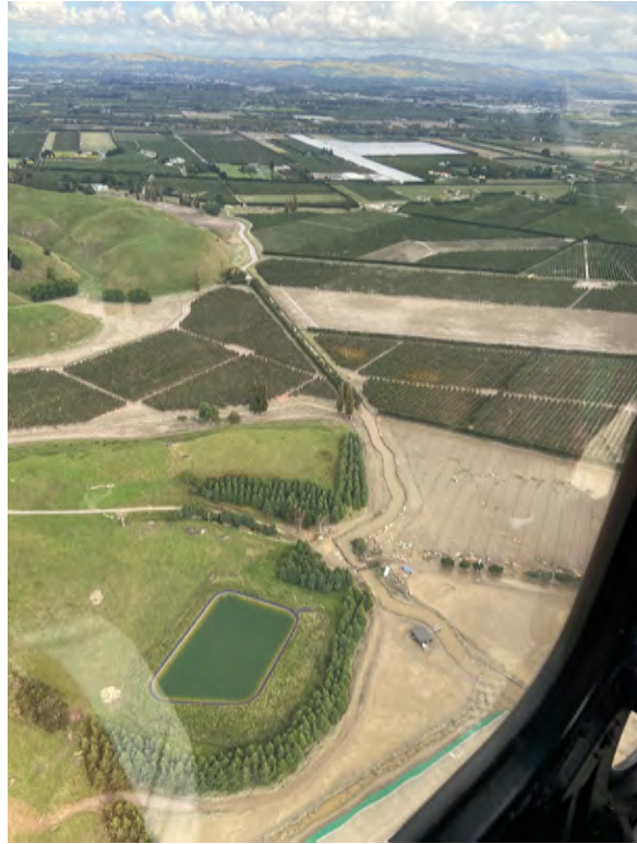
Photograph taken by our team from the helicopter on the way to Mahia, showing areas of flooding and silt
